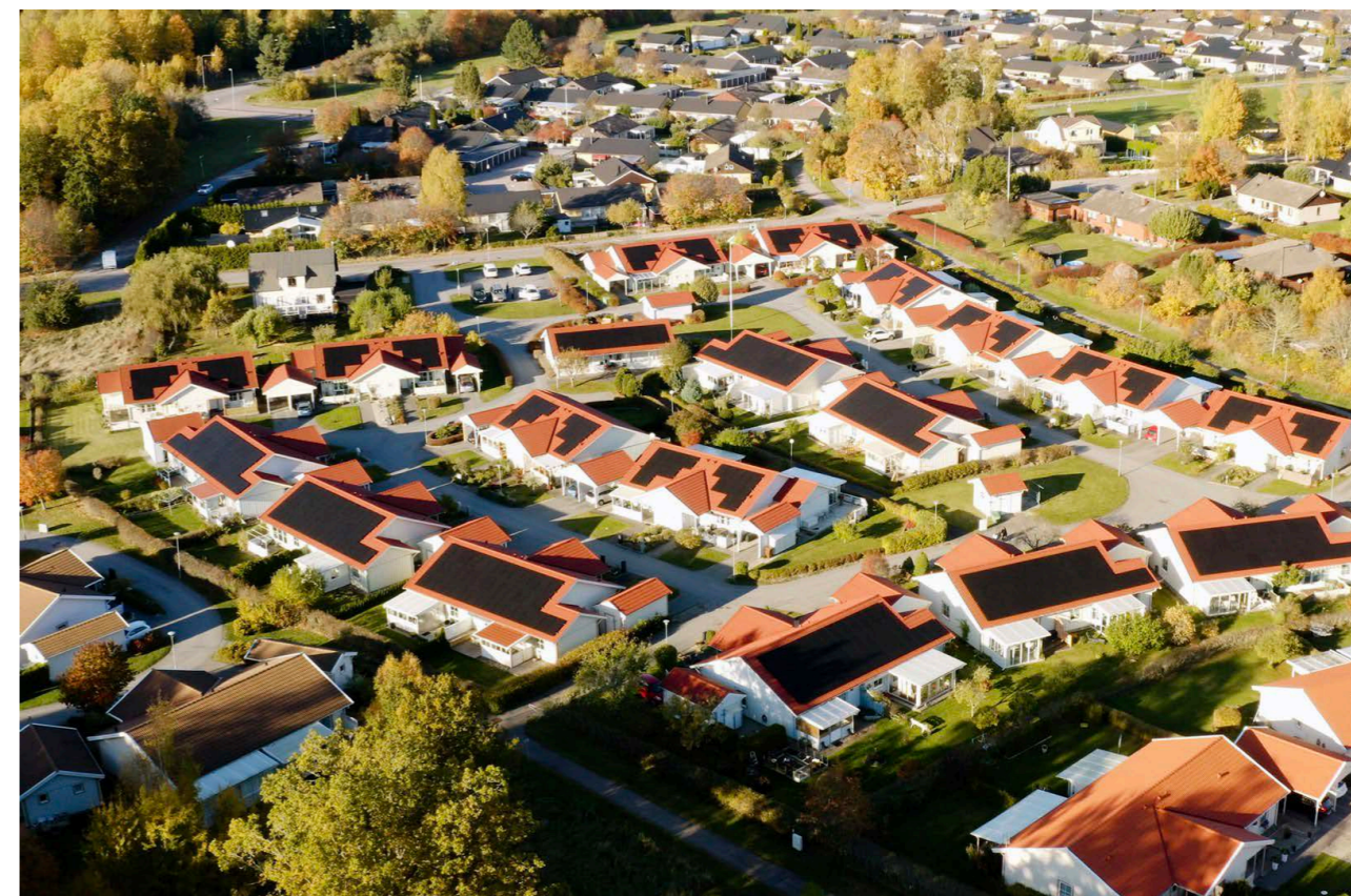
Remagruppen installed solar panels for BRF Mesta Hage in Eskilstuna, Sweden.
